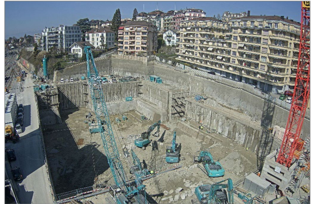
Elysée/mudac, Plateforme 10, Lausanne excavation supports
