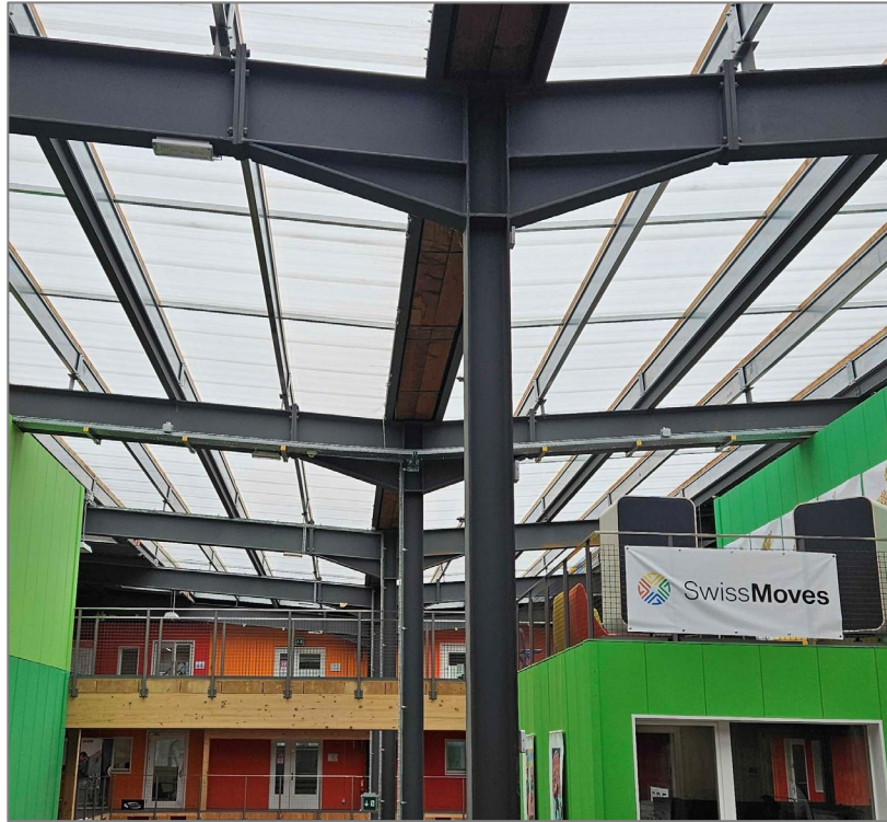
Halle Bleue, Blue Factory, Fribourg steel frame
